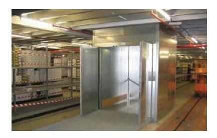
Most Goods Lifts rely on "call and send" controls on the landing, enabling the users to dispatch goods to other levels without stepping inside the lift car. However, should there be a site need to send a trained operative alongside the goods being moved, BKG have designed a special Goods Lift With Attendant. This enables the operative to travel with the goods and select which floor they need to travel to from within the lift car.
